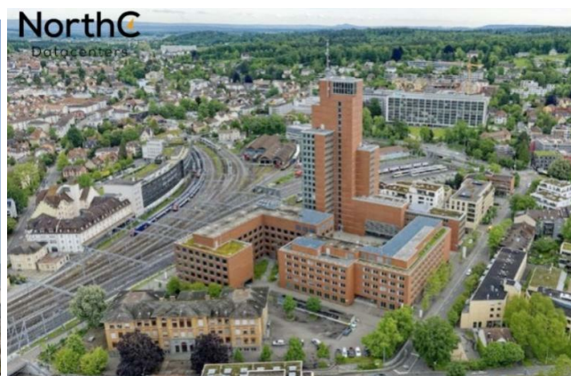
Abb: Rechenzentrum NorthC in Winterthur
